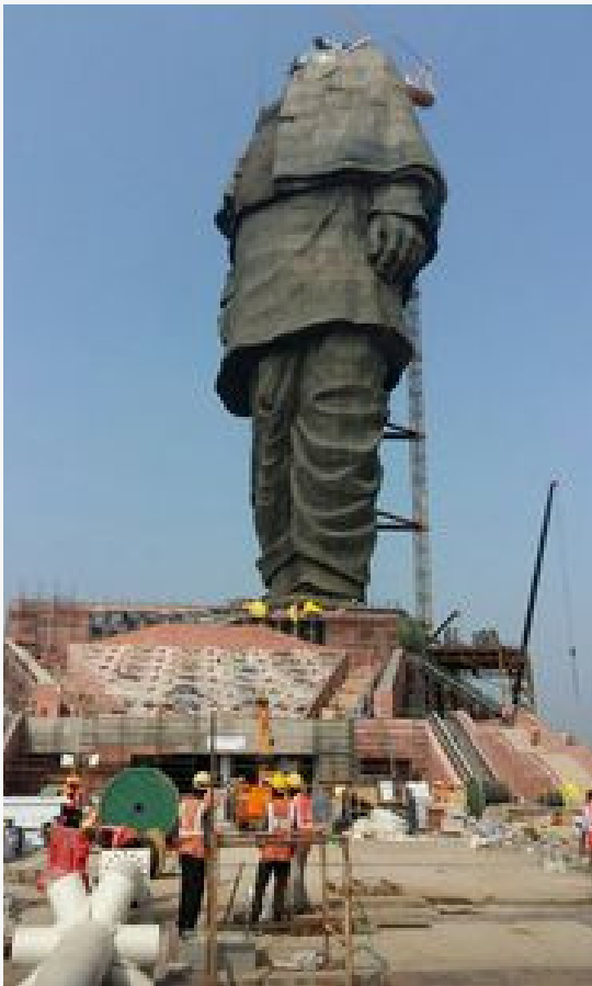
Fig: During the construction of : "Statue of Unity"
